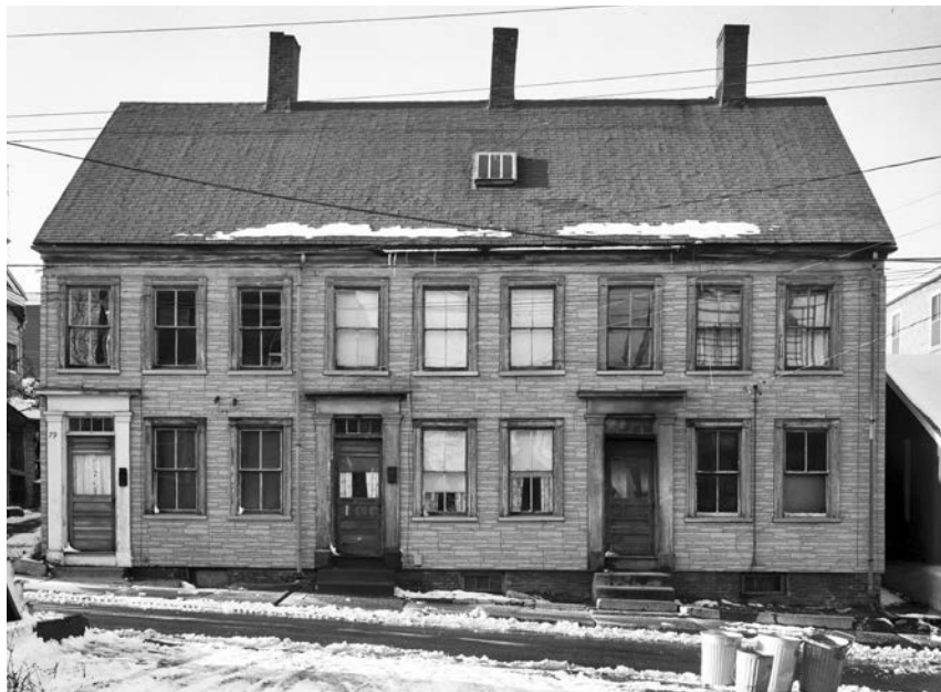
Multi-family house on Russell Street in the heart of the Italian North End in the 1960s, one of hundreds of buildings demolished by urban renewal. The building’s asphalt siding, a once-popular predecessor to aluminum and vinyl siding, was by this time considered cheap looking. Its frequent use gave the area a forlorn appearance. Courtesy of the Portsmouth Athenaeum.
