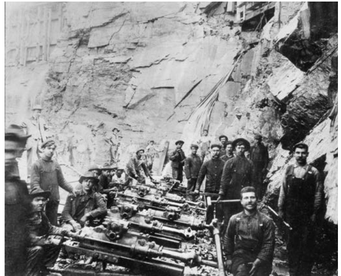
Workers with pneumatic drills prepare for the 1905 dynamiting of Henderson's Point, a hazard to navigation in the Piscataqua River. The Massachusetts company contracted to carry out the project brought Italian workers from Boston to Portsmouth to do the work. Courtesy of the Portsmouth Athenaeum.
